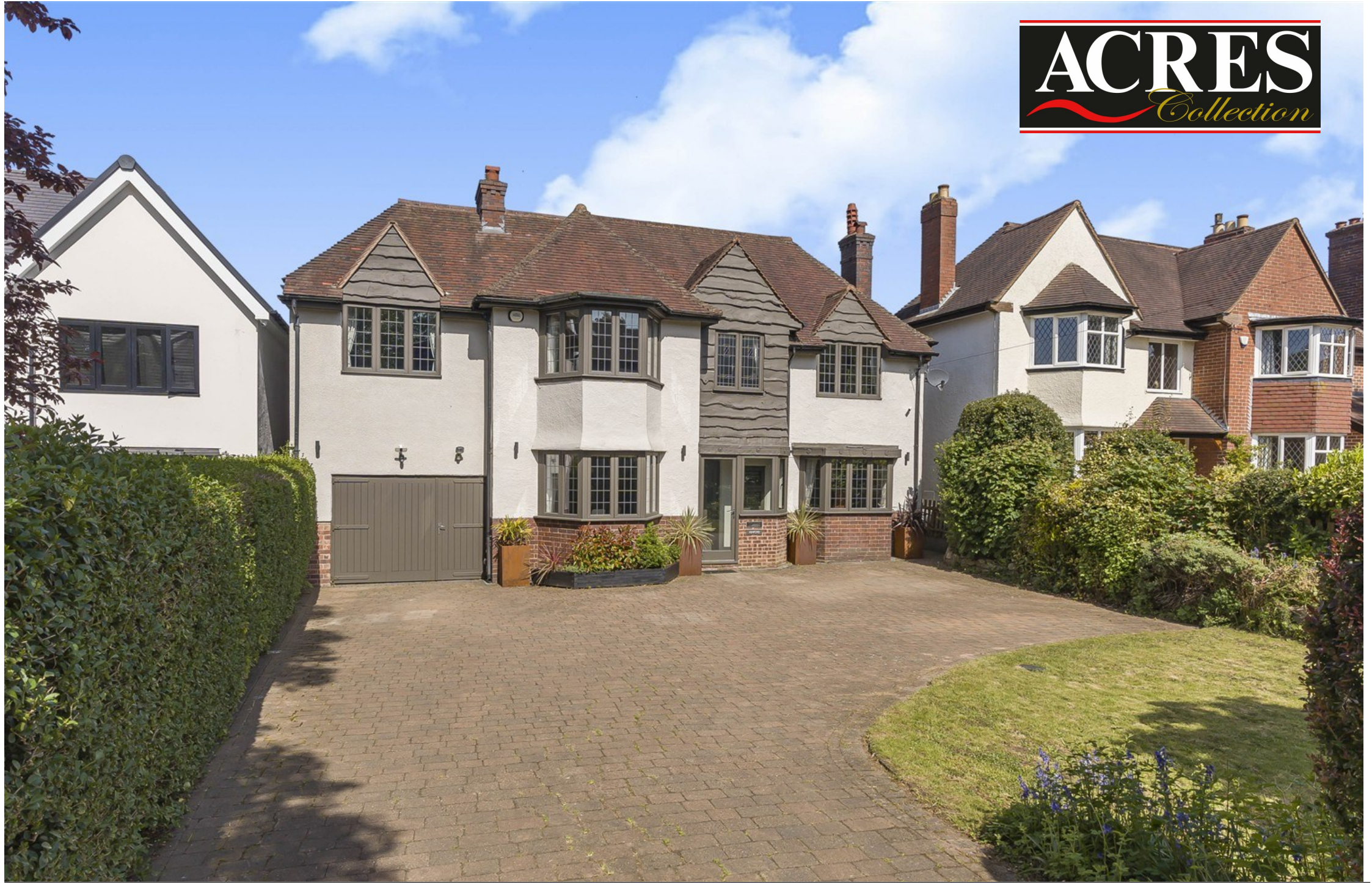
ASHFORD, 17 CROWN LANE, FOUR OAKS, B74 4SU
